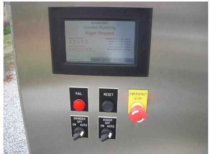
Figure 3 – Vendor provided HMIs and the Plant's SCADA HMI have to be developed to work together as part of the design and implementation process.
